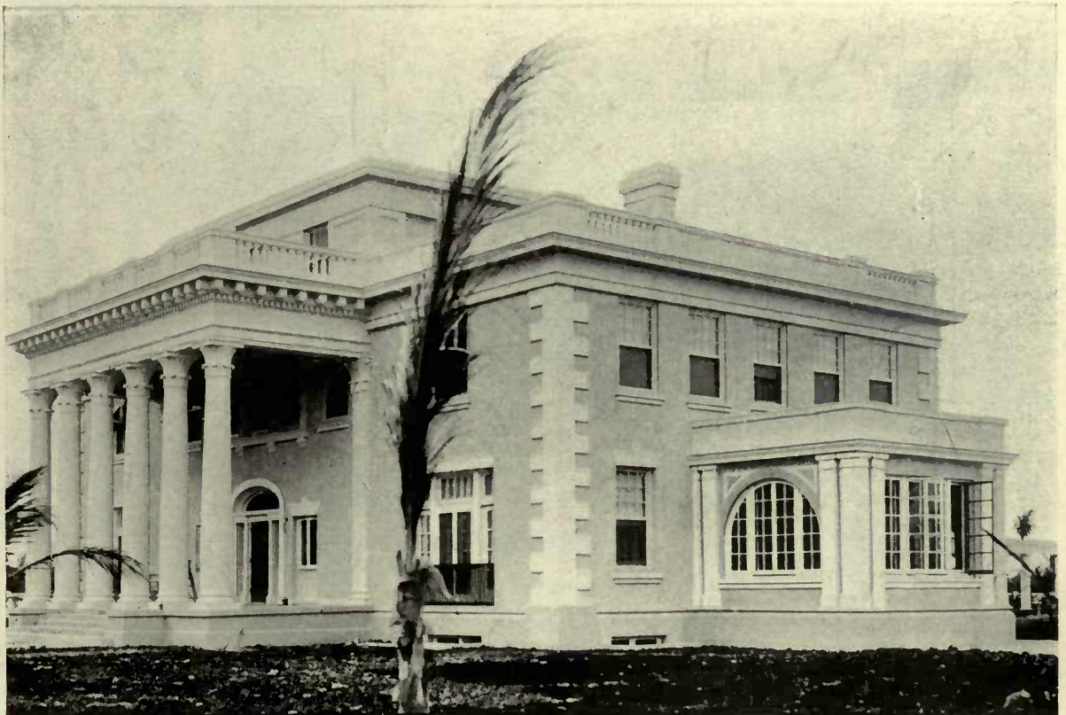
Hanna Residence, Miami, Florida. August Geiger, Architect, J. B. Orr, Stucco Contractor All stucco waterproofed with Truscon Waterproofing Paste, Concentrated .
